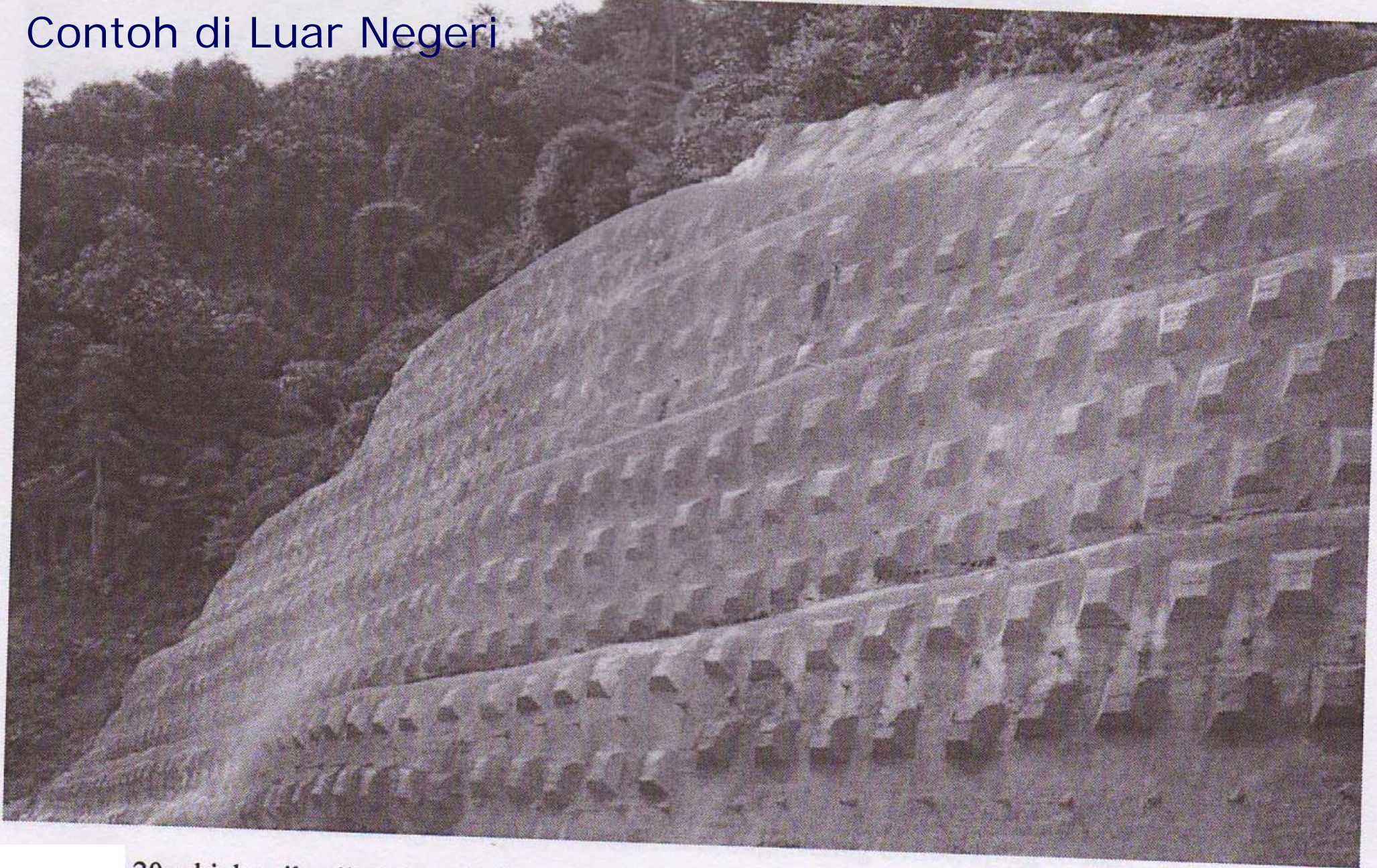
20m high soil nailed slope in Kuala Lumpur.
