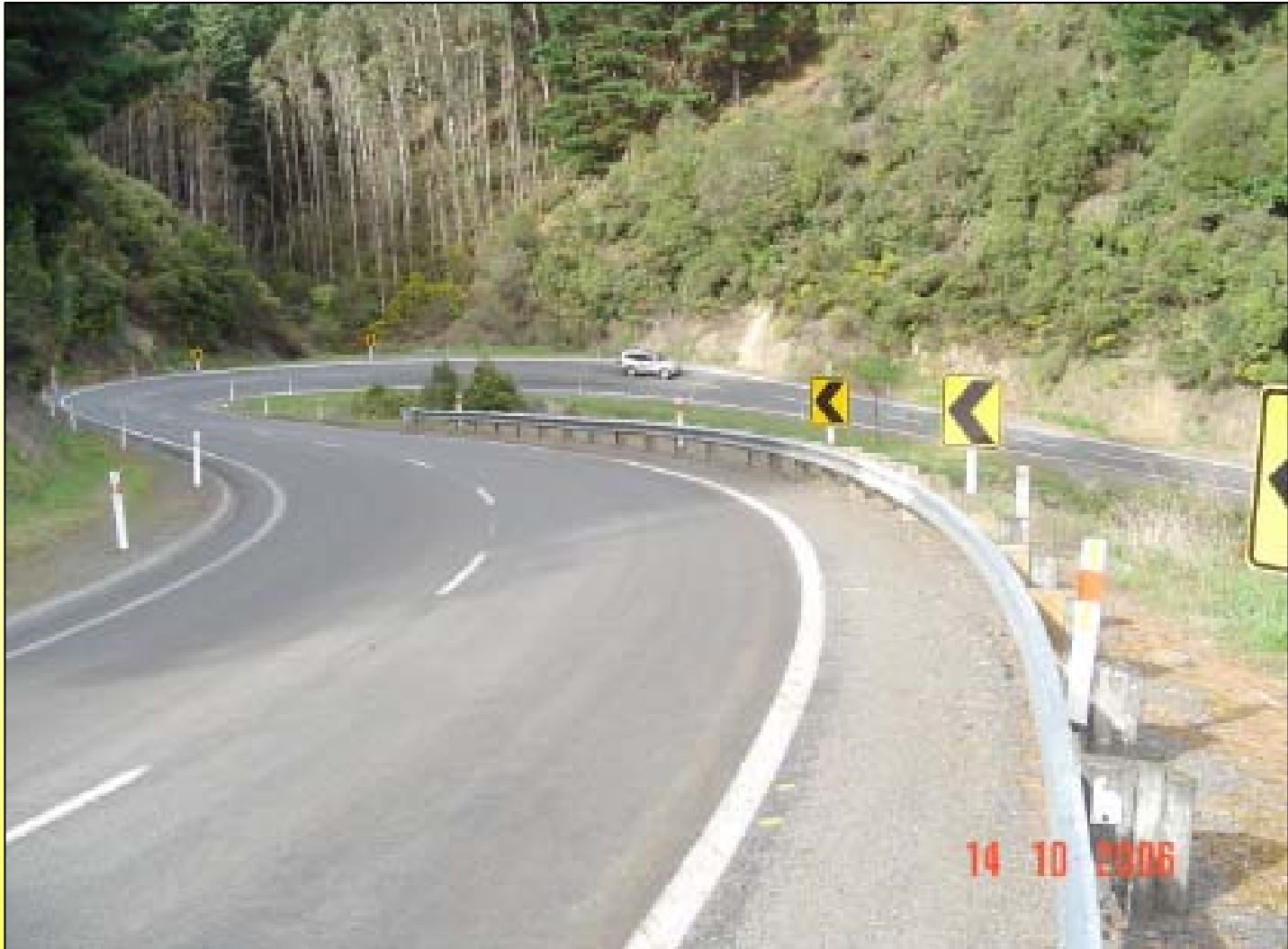
Chip Seal – in New Zealand
