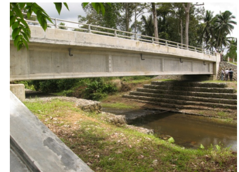
Gelagar Beton Pratekan (20m)
