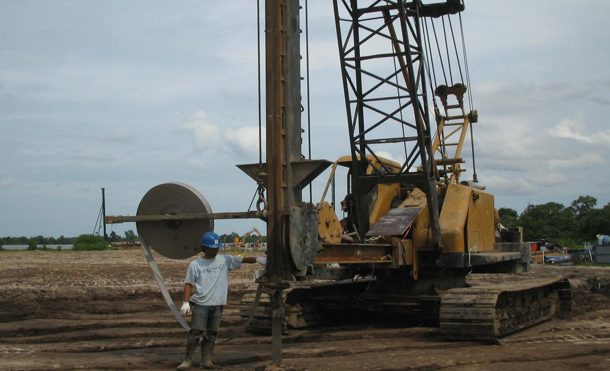
TRIAL PEMASANGAN VERTICAL DRAIN
