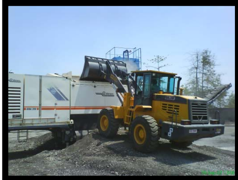
Pengisian Material (RAP + Agregat)
